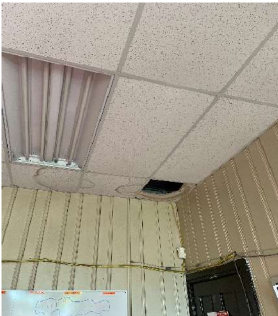
Figure 9: Missing ceiling tiles and water stains
