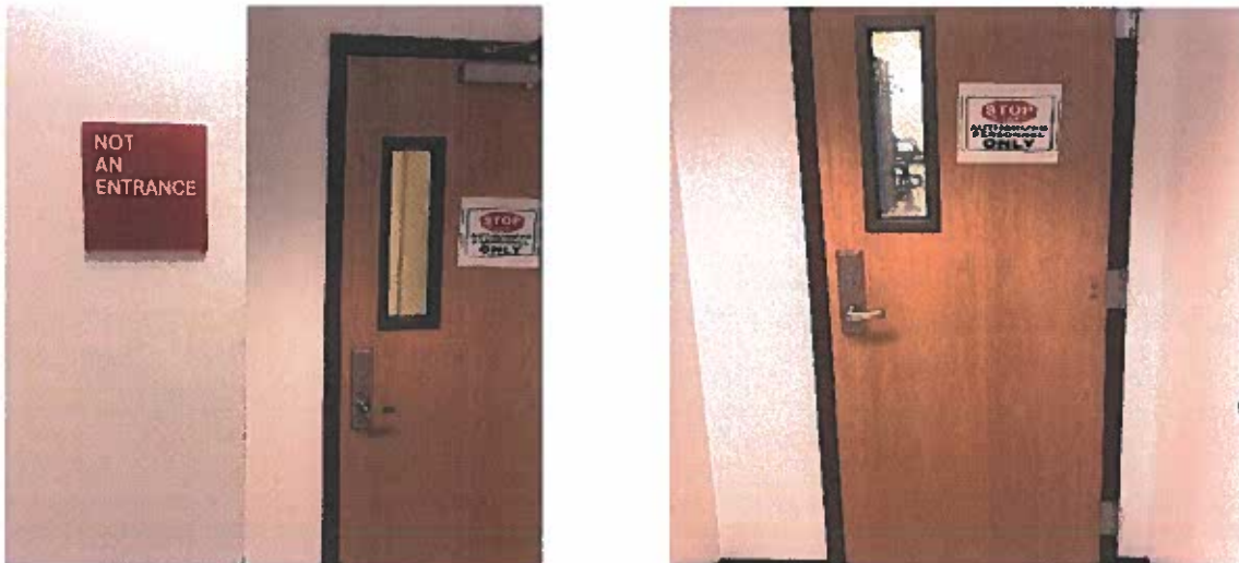
Figure 10: Access door repaired and secured (July 2022)
