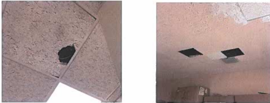
Figure 7: Damaged ceiling tiles
