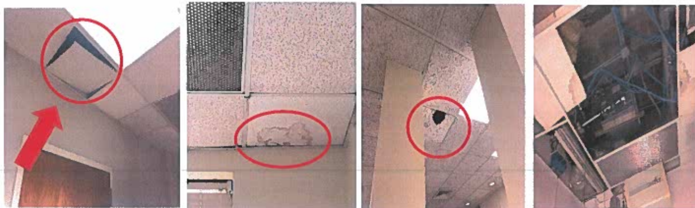
Figure 4: Unsecured and damaged access door
