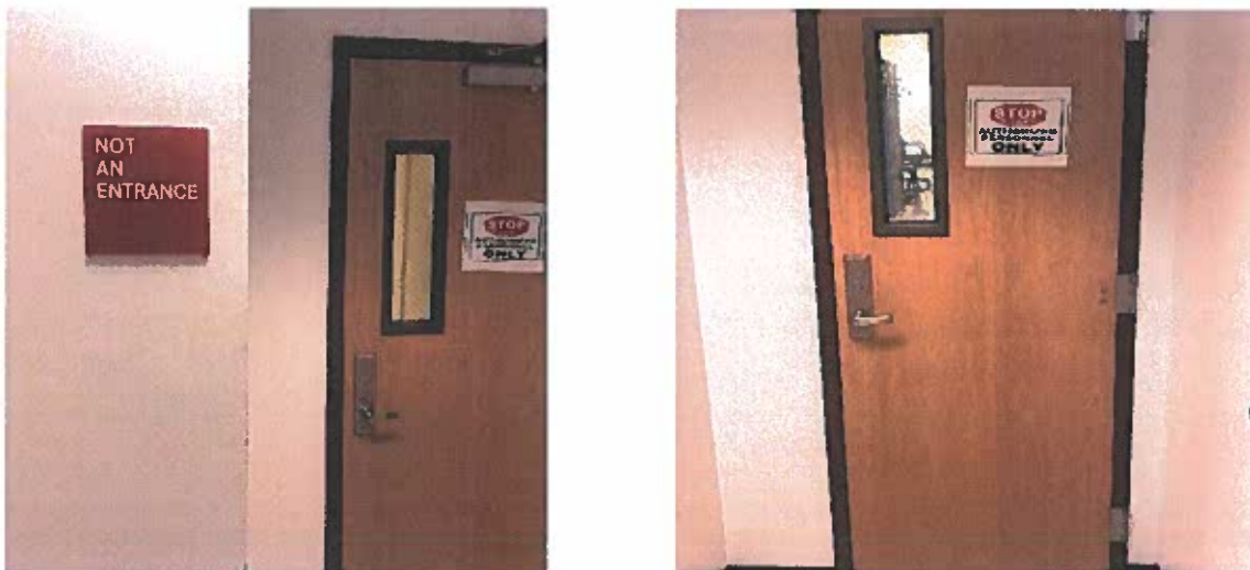
Figure 10: Access door repaired and secured (July 2022)
