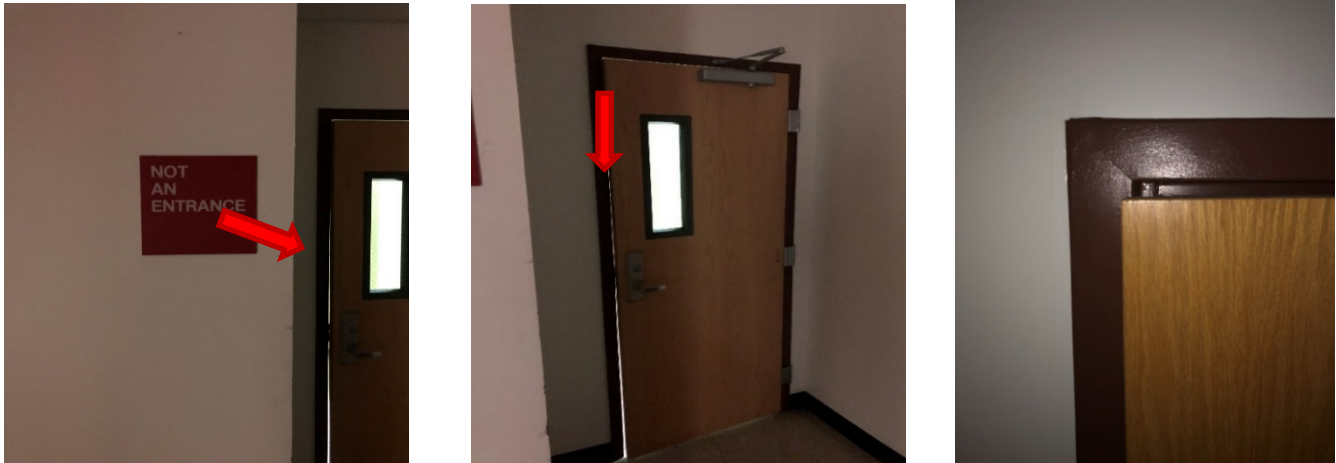
Figure 4: Unsecured and damaged access door
