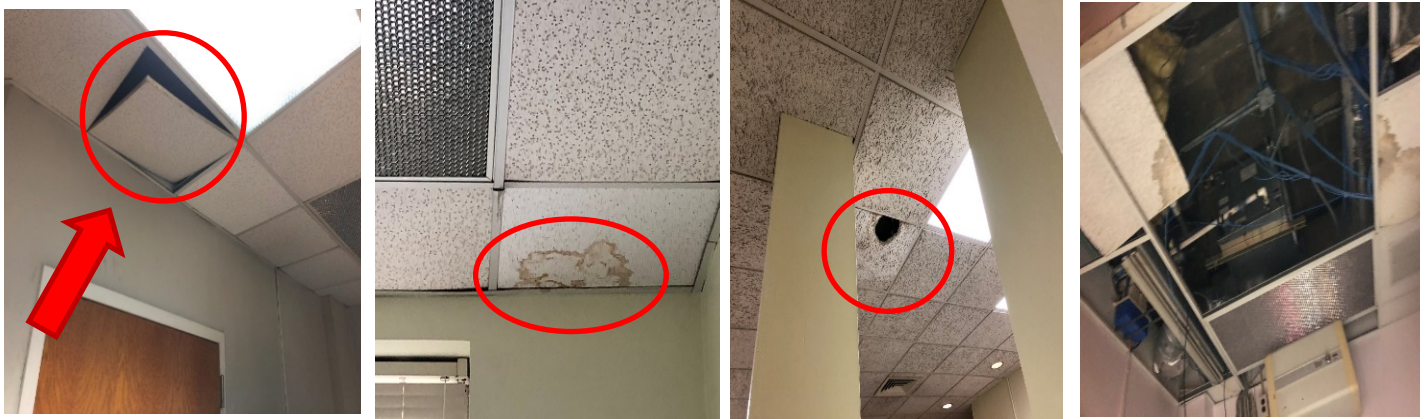
Figure 4: Unsecured and damaged access door
